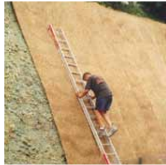
GREENFIX Rockmat Type 5D dengimas ant 65° statumo šlaito
